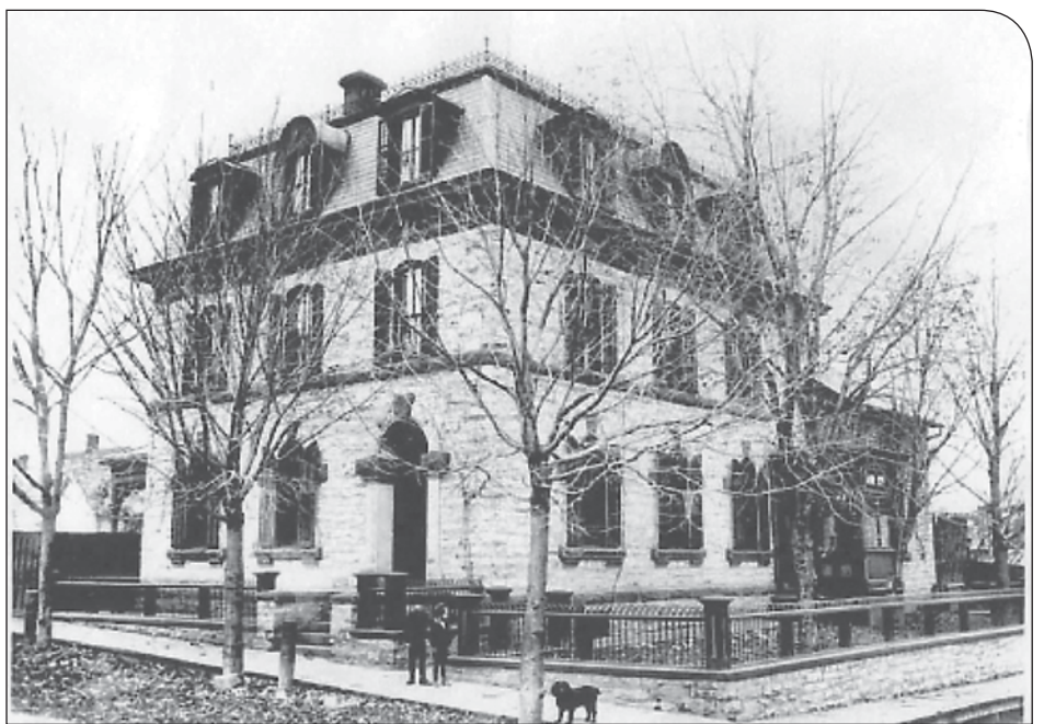
The Almonte Legion as it appeared prior to the fire that destroyed its third floor
